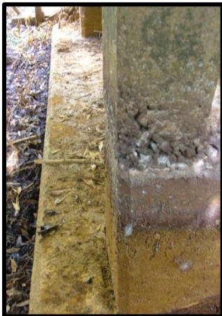
Concrete cancer from acid waters.
