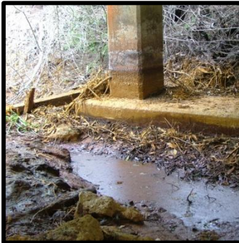
Concrete cancer from acid waters.
